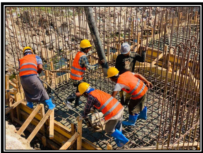
Restoration of Damaged Bridge
