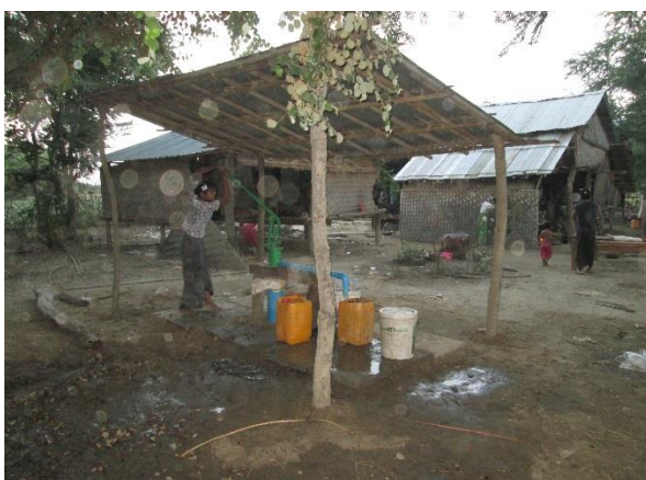
Elevated Tube well in flooding affected village of Yenanchaung Township
