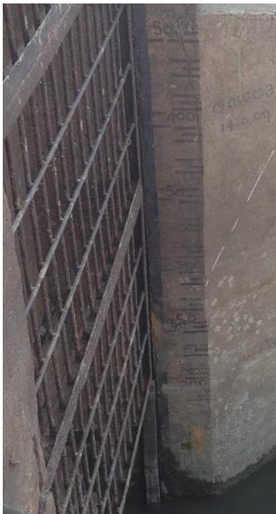
Figures 16, 17 & 18: Show how difficult it is to obtain accurate gauge readings
