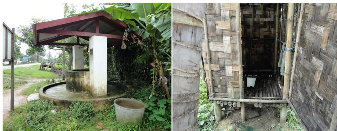
Brick lined Dug well with roofing (ECHO)
