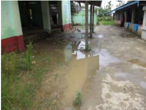
Figure 28 Poor water drainage in schools
