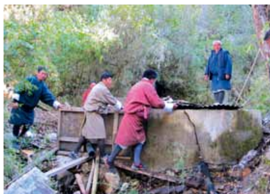
As part of the improvement plan, the damaged wall on an existing intake tank (right) is being repaired, and a supplementary intake tank is under construction (left) in Dhaji, Bhutan
