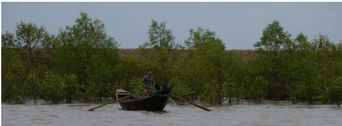
Figure 4-13 Polder dyke in the background built very close to the mangrove shore, the mangroves lose their required size of habitat and will eventually perish.
