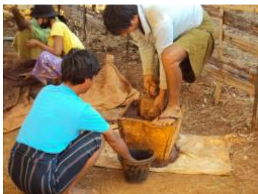
Pictures 3 & 4: Demonstration of construction of fuel efficient clay stove using local materials (left); Fuel efficient clay stoves are dried indoors (right)
