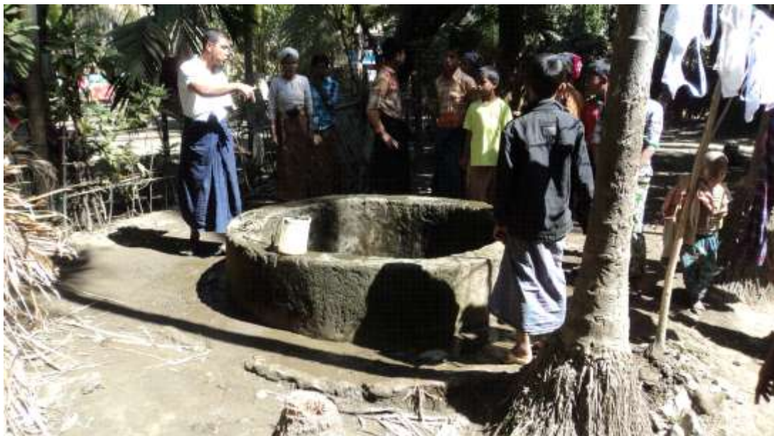
Fig. 20: Existing water well
