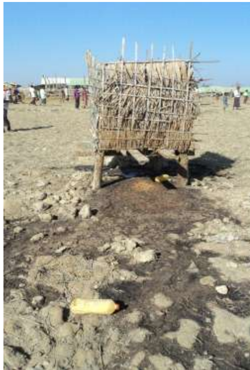
Fig. 18: Abandoned latrines need to be decommissioned before wet season
