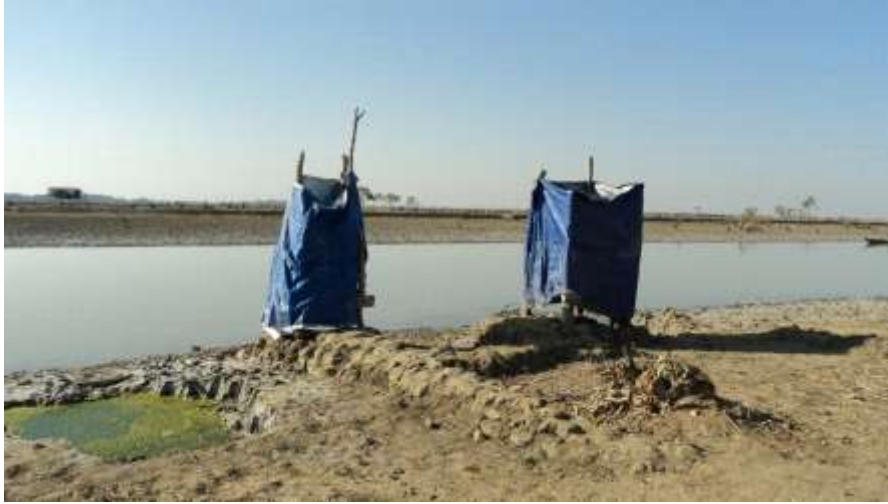
Fig. 17: Pan-PVC pipe latrines discharging into the river
