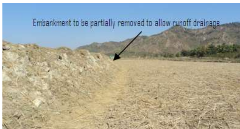
Fig. 22: Embankment in the West side of the paddy field
