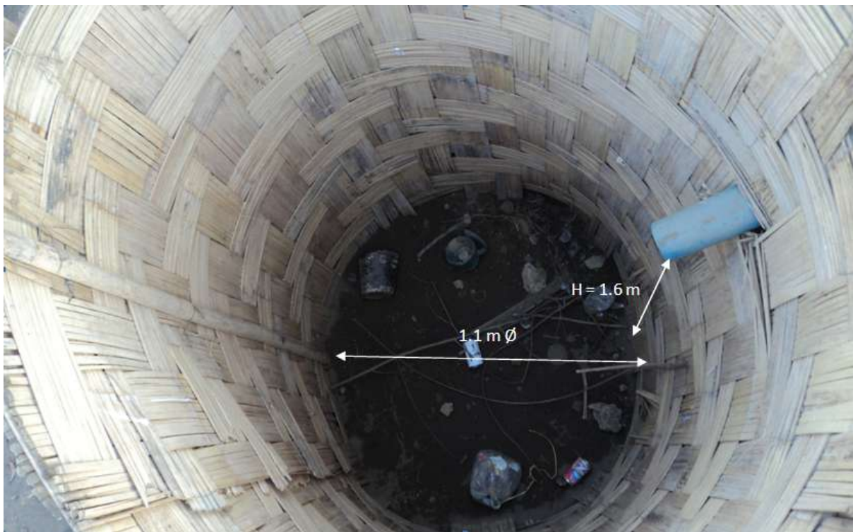
Fig. 11: Double bamboo lined pit latrine
