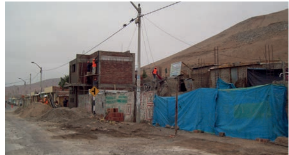
Figure 6. Construction in Ite, Peru
