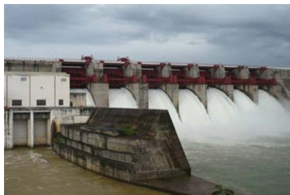
Sedawgyi Hydropower Station
