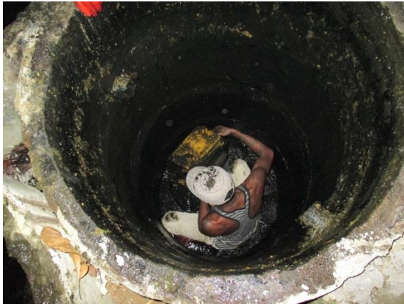
Tank bottom desludging...
