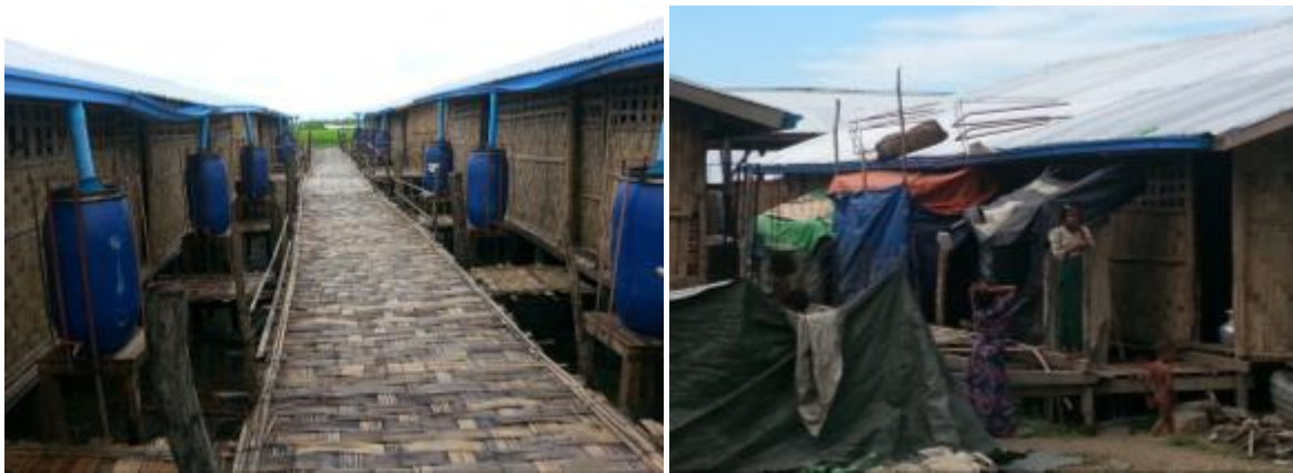
Figure 2 – RWHS just installed and some days after the end of the rainy season
