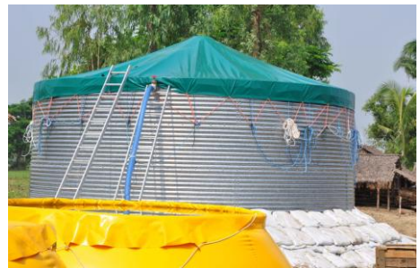
Figure 6: Tank for water storage (50m 3 )
