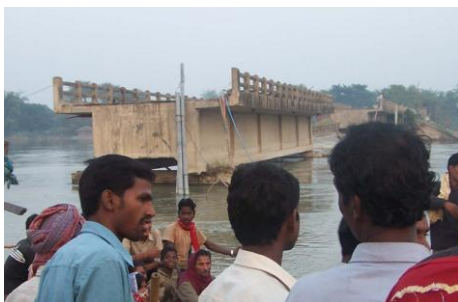
Figure 1: Rupture of transport and communication services (Bihar, 2009)
