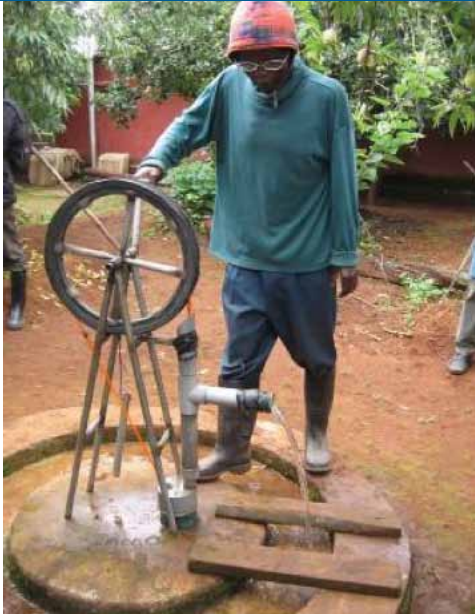
A Tube recharge system installed for a family in Njombe in Tanzania in 2011
