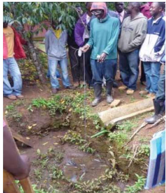
When the cloth filter is dirty it is cleaned by lifting and shaking it. Before the Tube recharge, this well dried up for 2 months every year. Since 2011 the well has water all year round. The water is used for 1 cow, a family of 6 persons and irrigation of a garden of 300 m 2
