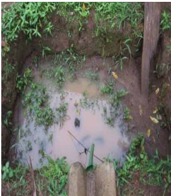
Whenever it rains the pit fills up and water infiltrates to the ground via a cloth filter and a sand filter
