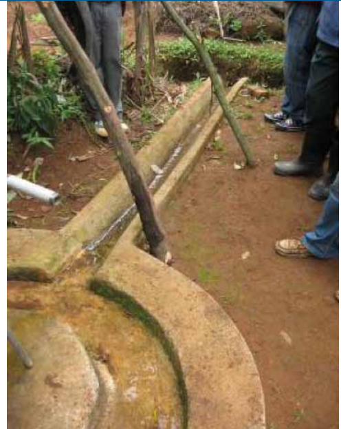
The water from the roof and run off water from the area around the house is led to the pit.
