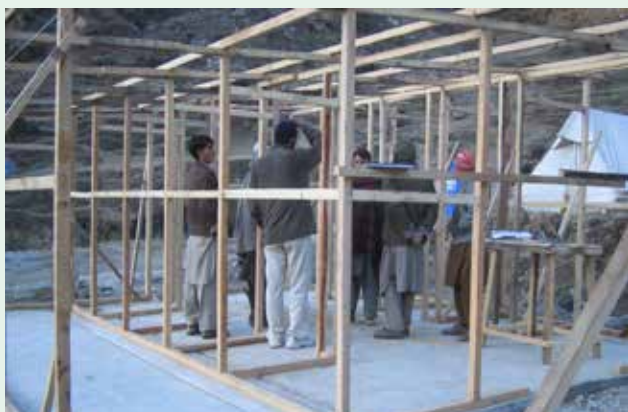
Warm bathing unit under construction – laundry area seen to the left of the picture
