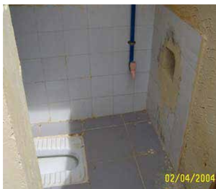
Disposal shoot inside the latrine
