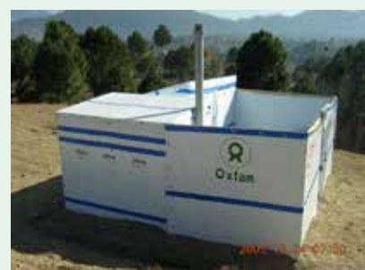
Screened latrine and bathing unit
