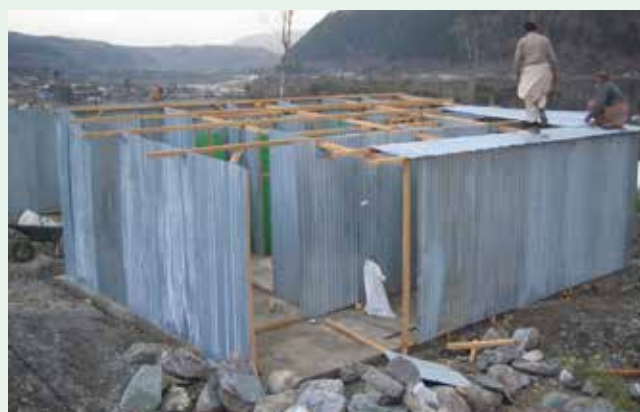
Warm bathing unit under construction – laundry area seen to the front and right of the picture
