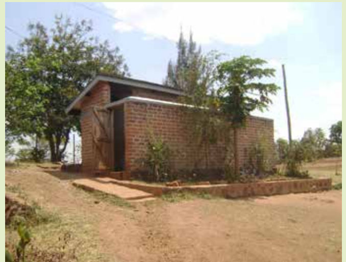
Example of a well-designed latrine with privacy wall
