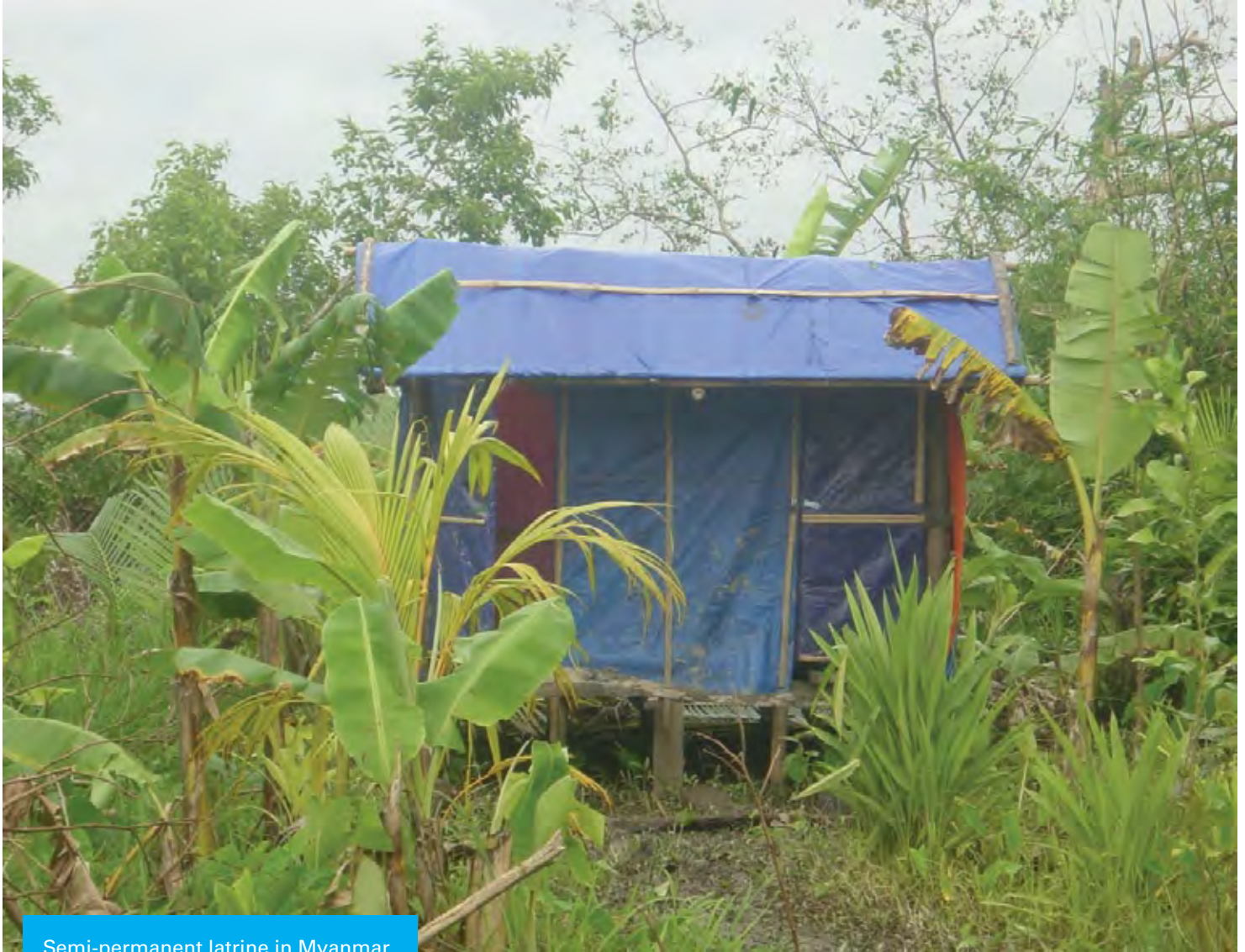
Semi-permanent latrine in Myanmar
