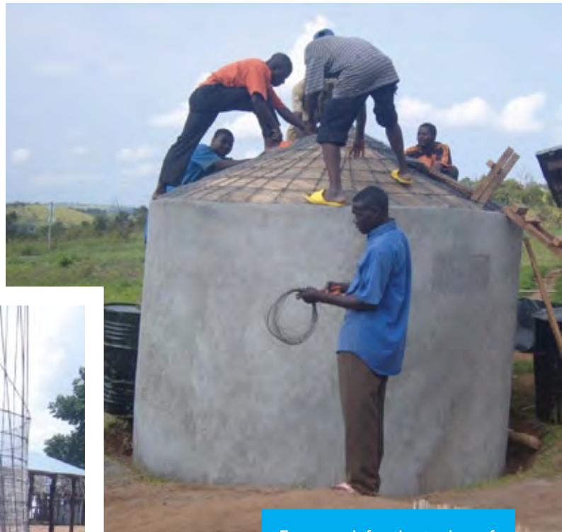
Formwork for the tank roof
