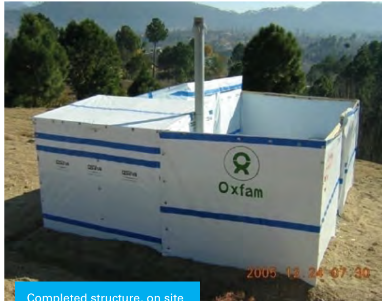
Completed structure, on site
