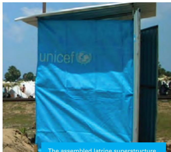
The assembled latrine superstructure
