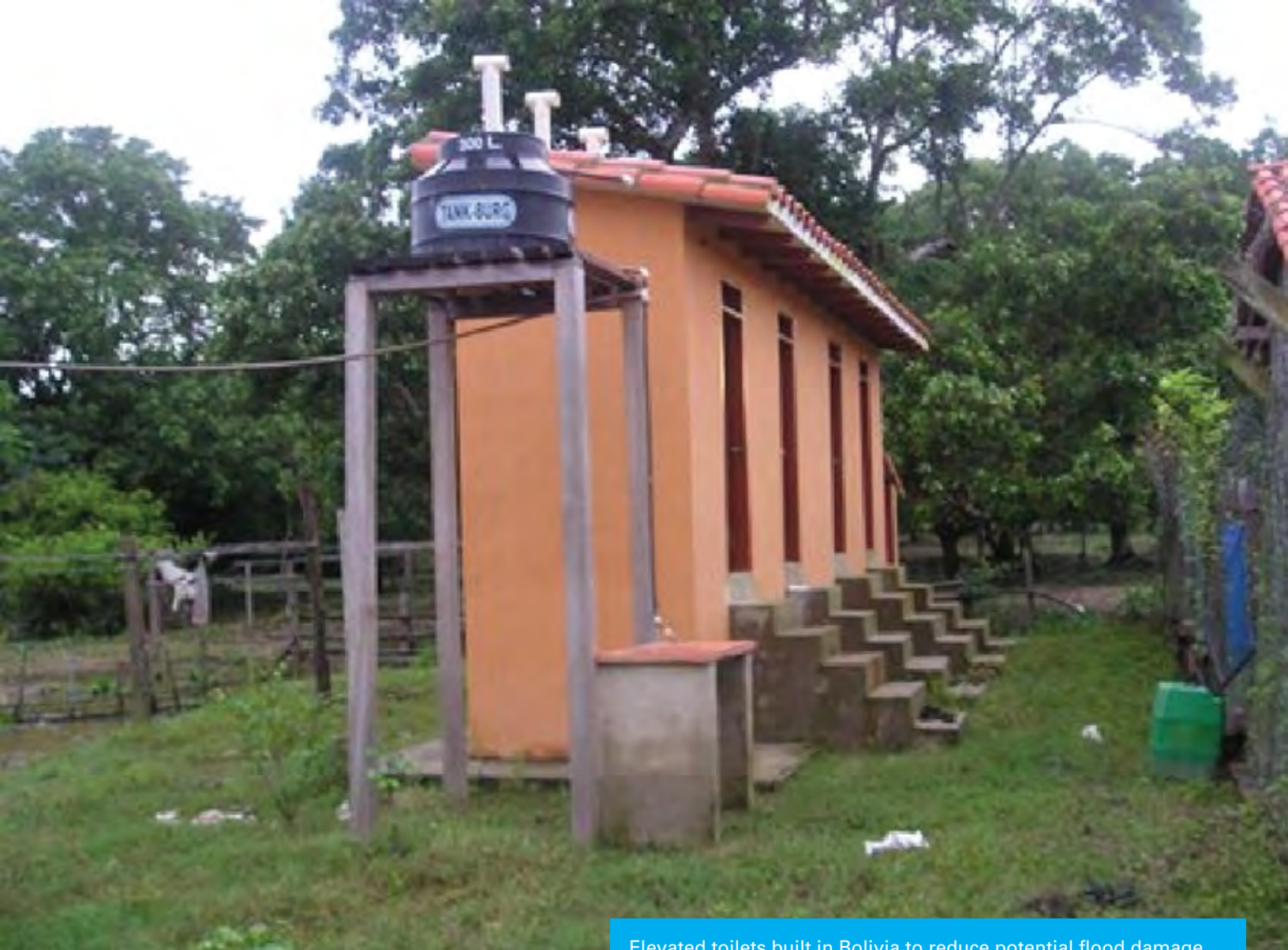
Elevated toilets built in Bolivia to reduce potential flood damage
