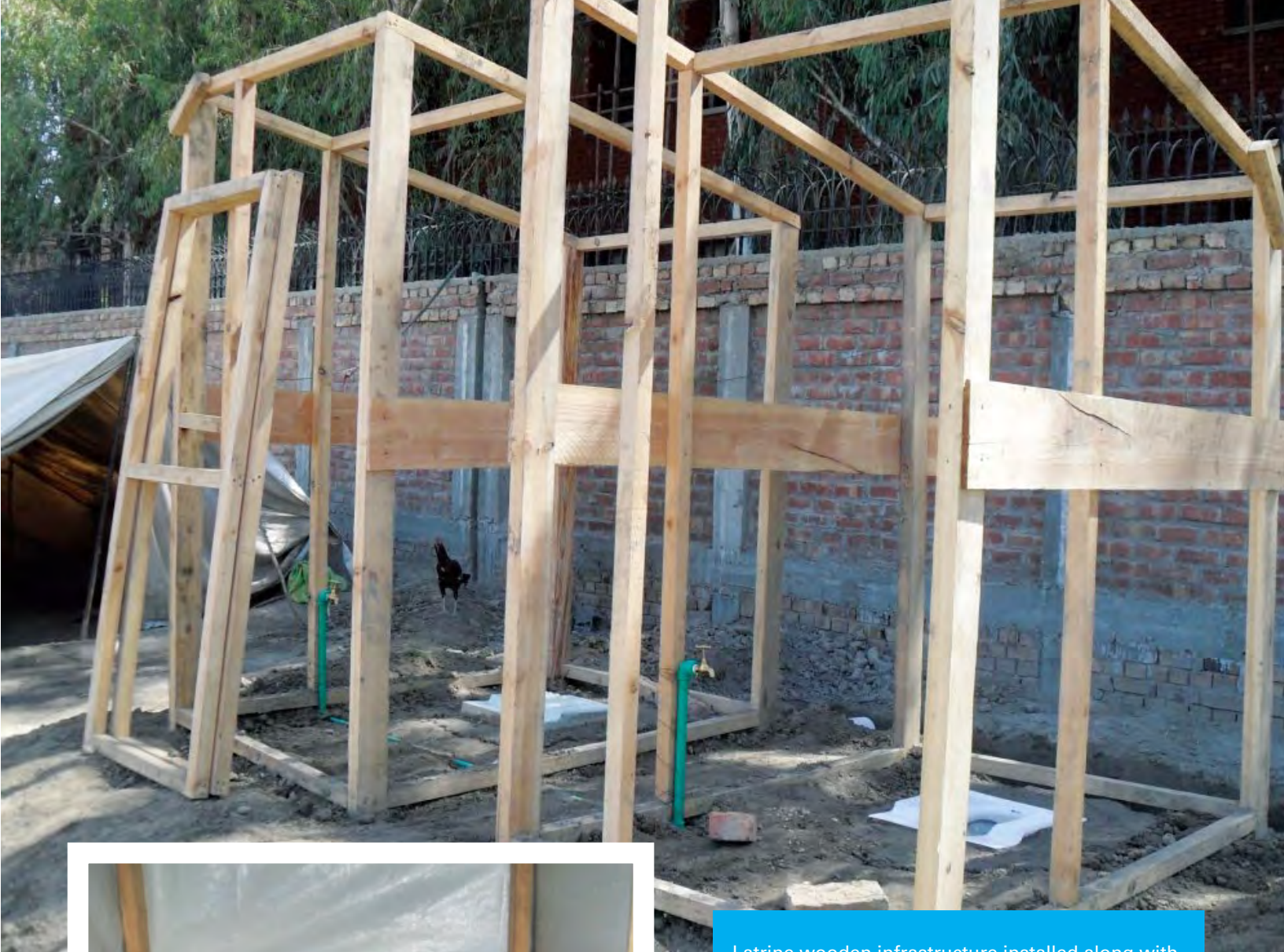
Latrine wooden infrastructure installed along with pour flush pans (above) and completed latrine with plastic sheeting walls (left)
