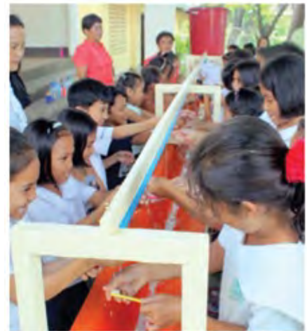
The punched pipe hand-washing system, which allows many children to wash their hands at the same time, was developed by the Fit for School organization in the Philippines.
