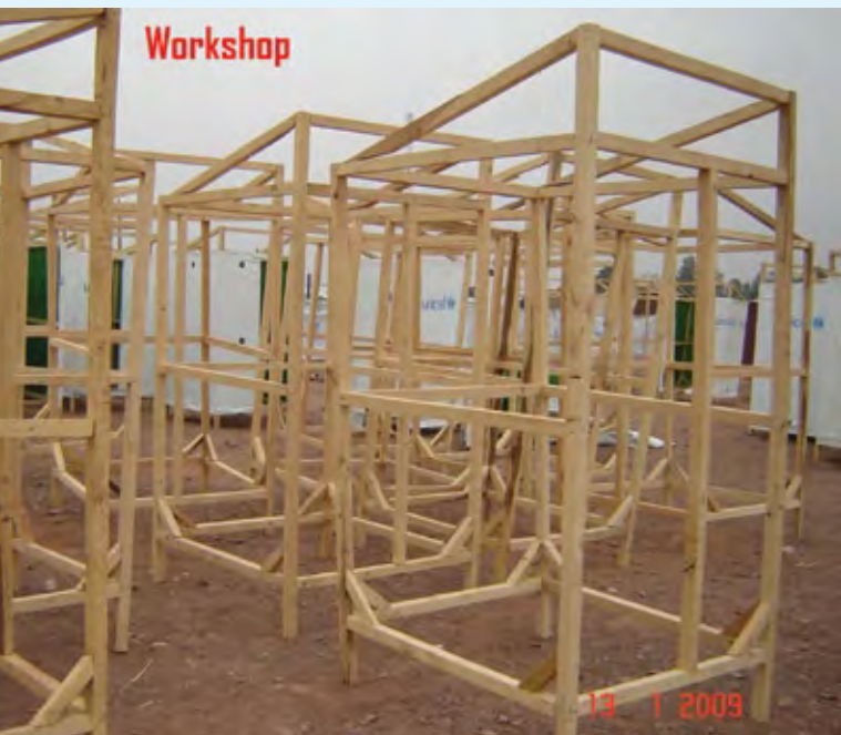
Latrine superstructures are prefabricated in a central yard and moved to the required location when pits are dug (left). At right, a teacher demonstrates hand washing with children in a temporary learning space.
