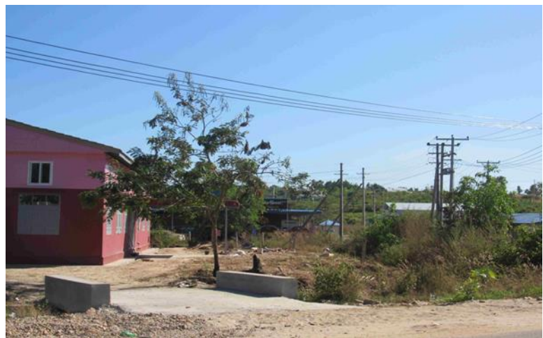
Figure 17 Enterprise in Industrial Zone
