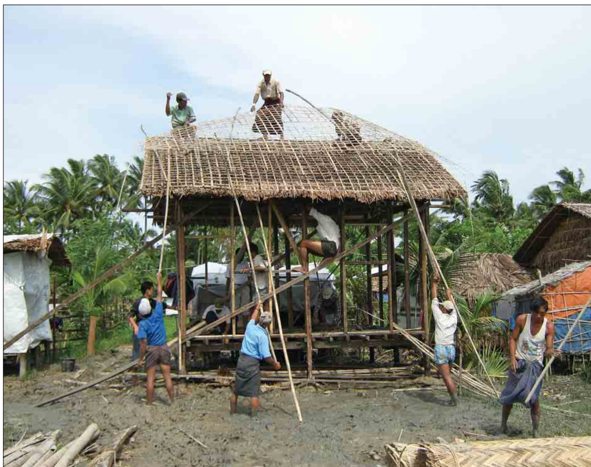
Covering bamboo canopy(Kyet-nin) over the roof ▲
