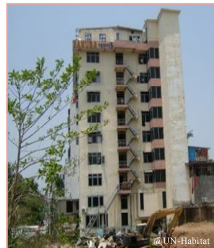
Fire escape ladder system in a high-rise building
