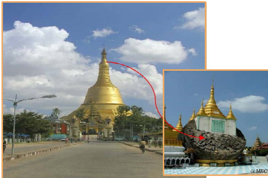
Top portion of Shwe Maw Daw Pagoda fallen down at the banana bud portion by 1917 Bago Earthquake. Fortunately, it was not crushed. Small pagoda was built on top of it later.
