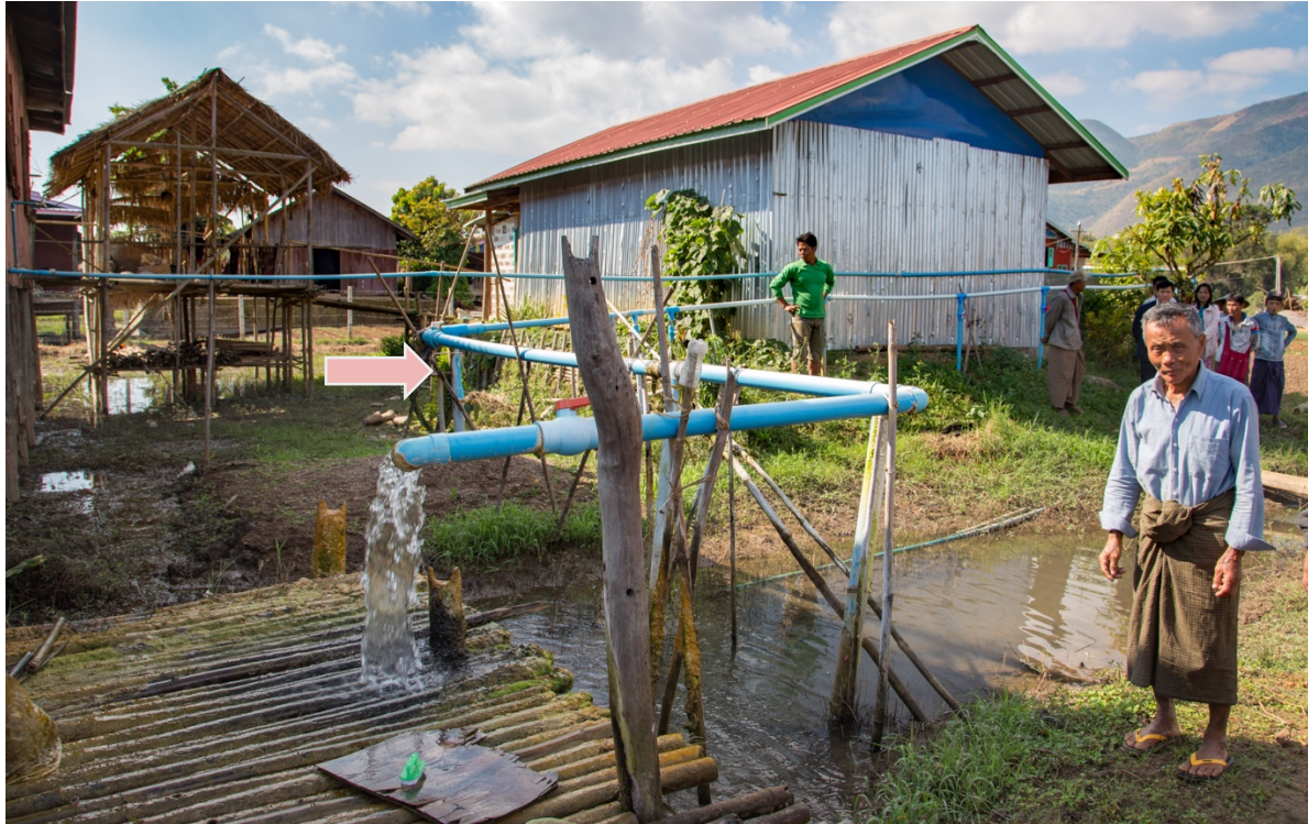
Figure 22: Nyaungshwe township, Taung Poet Gyi village. An artesian well, roughly 320ft deep, flows year-round into a canal as the construction is unable to contain the pressure if the valves are closed. Following this early 'lucky find' households tried a further 10 deep tubewells, with five failing, four providing a low quantity of water and one having a higher yield, but none were artesian. No other artesian wells were found during the field visits.
