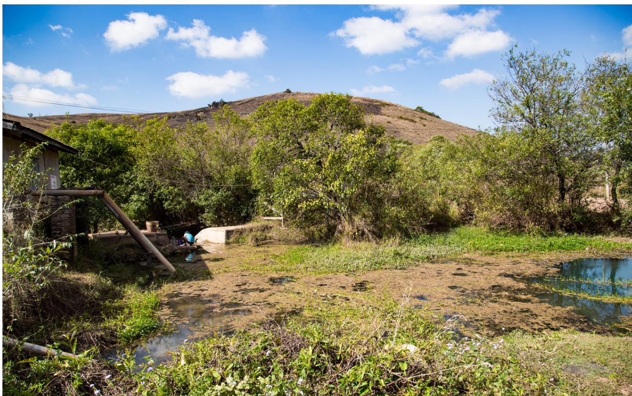
Figure 8: Kalaw Township, Ong Ywar Ma village. Shallow natural spring with numerous spring holes under and around the pond, created by a DRD built dam which overflows into a stream.
