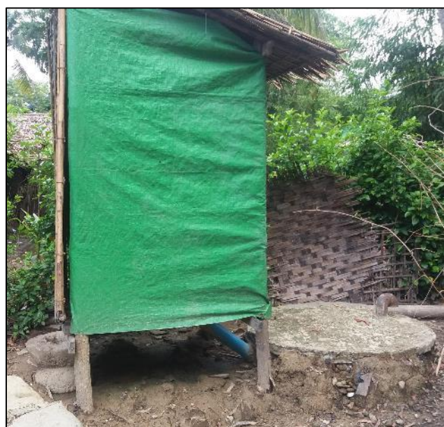
Household offset concrete pit latrine built by community members in Rathedaung CLTS site
